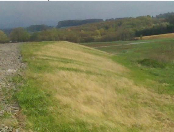
Well Pad Embankment
